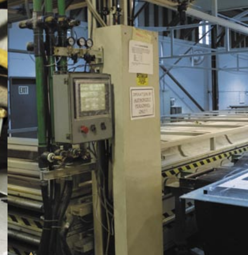
Cradled in vacuum pouches, Country Coach walls, floors, and roofs are laminated under 4psi of pressure for at least one hour.
