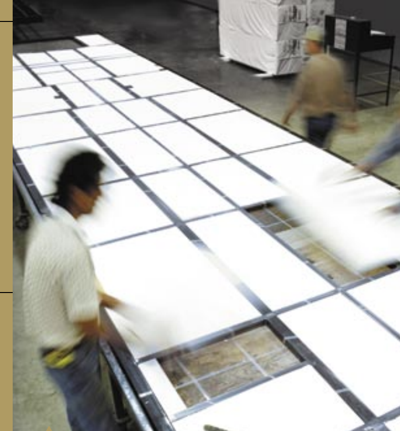
High-density styrene insulation is hand-fitted to the steel walls, floor, and roof of each motorcoach.
