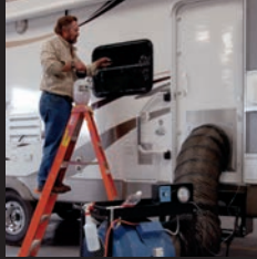
Seal Tech Air Pressure Test
