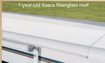
1-year-old Itasca fiberglass roof
