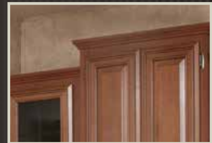
Raised panel cabinet doors with crowned molding found in the kitchen.
